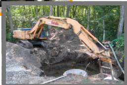
Installing a Geo-Thermal Heating System
