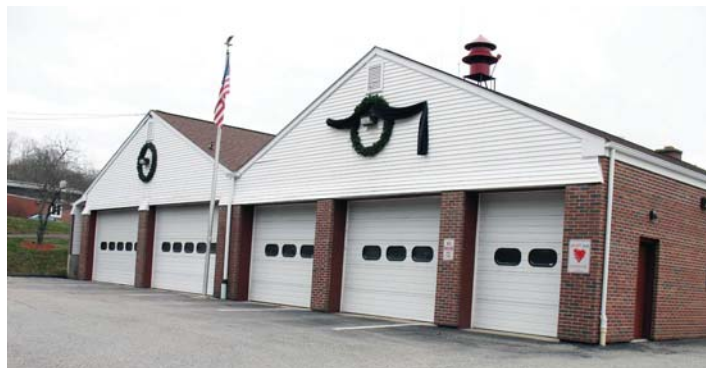
The Volunteer Fire Station Building is experiencing space shortages.
