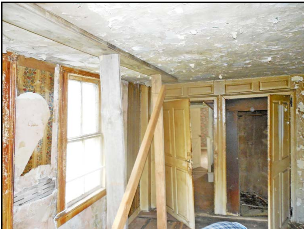
Photo P08 – Shoring of 2 nd floor joists at south/front wall.
